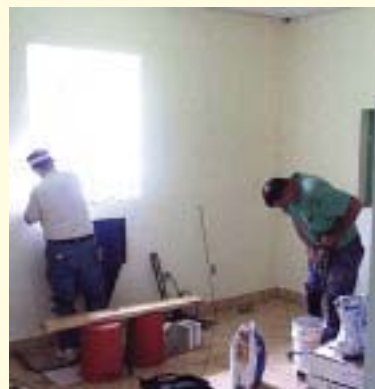
Preparing the walls for painting at the seminary.
