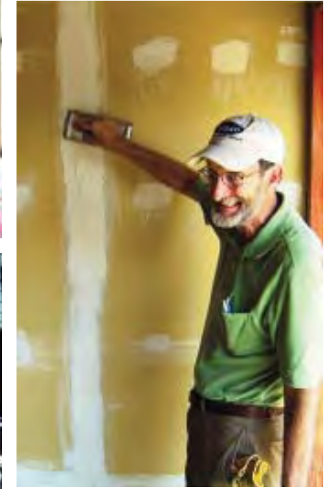
Author and drywaller, Kevin Verett, making repairs at Ogima's home.
