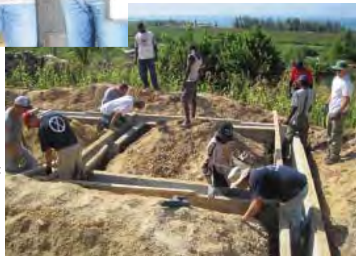
Glace team begins construction on a new Home for Haiti.
