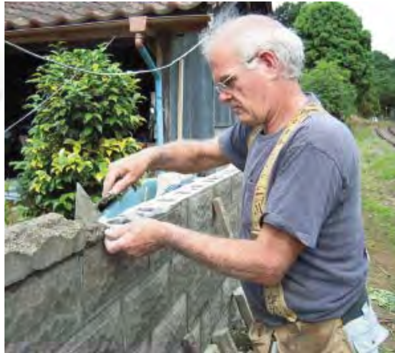
OMS missionary, Steve King, repairing earthquake damage.
